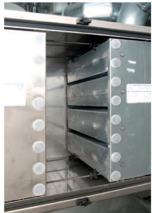
Purification filters for intake-air
