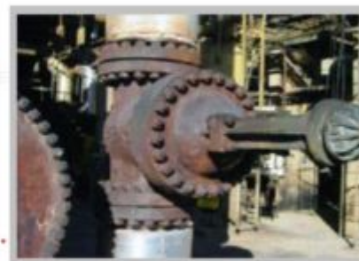
Insulate all thermal bridges like for example valves
